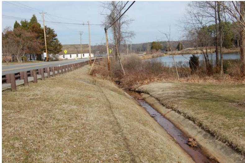
Picture 2: Concrete Swale across from the Post Office
