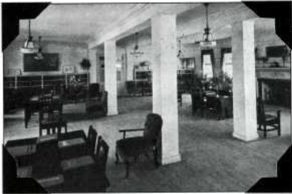
With the furniture removed, this became the ballroom for dances at Charlotte Hall.
