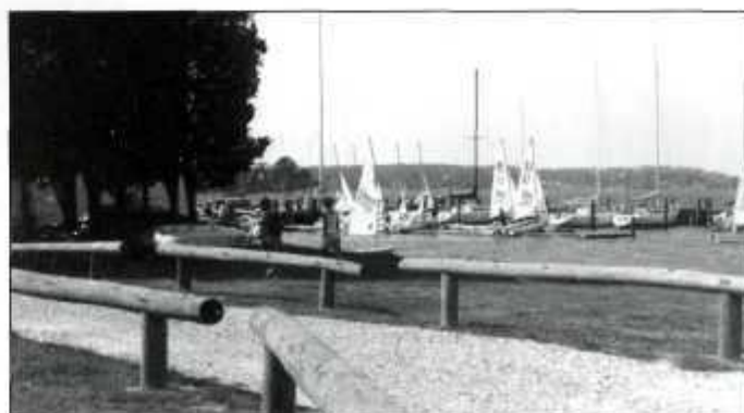
The Waterfront—the College's natural wonder—as it begins renovation.
