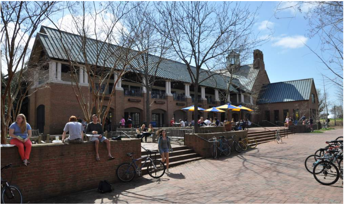
2000 Campus Center renovation and expansion
