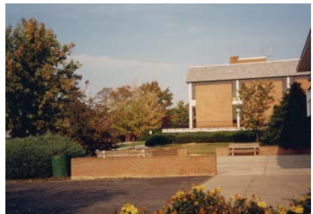
Library Prior to Renovation
