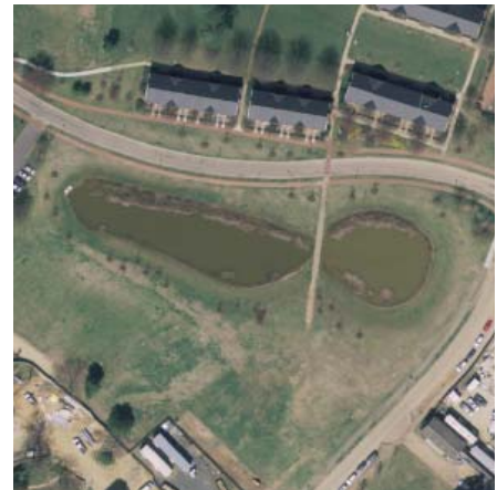
Figure 14. Aerial view of stormwater pond
