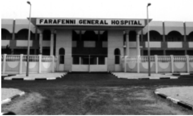
The new hospital at Farafenni is not yet operational.
