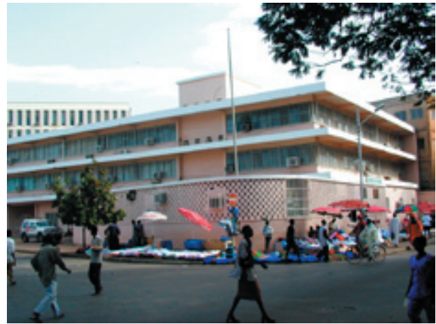
The Bedford building has a long history. Currently it houses the Department of State for Education.
