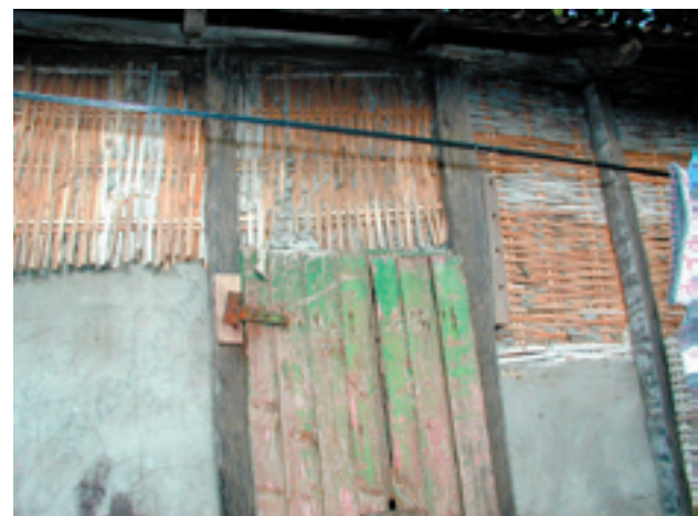
Close-up of Krinting House showing the bamboo and wattle construction.
