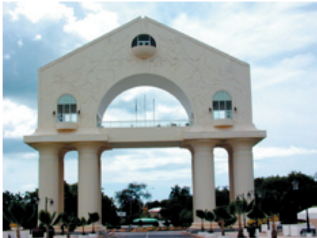
Looking at Arch 22 from the Banjul side of Independence Drive.
